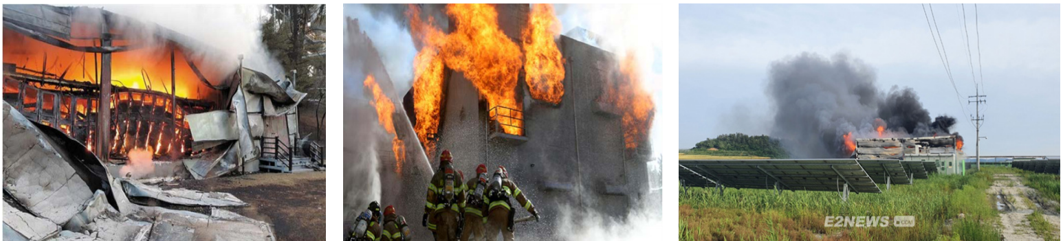
Figure 23. A series of 29 Lithium-ion BESS fires occurred in South Korea from 2017–2019. (IMIA Report and E2 News Photo)
