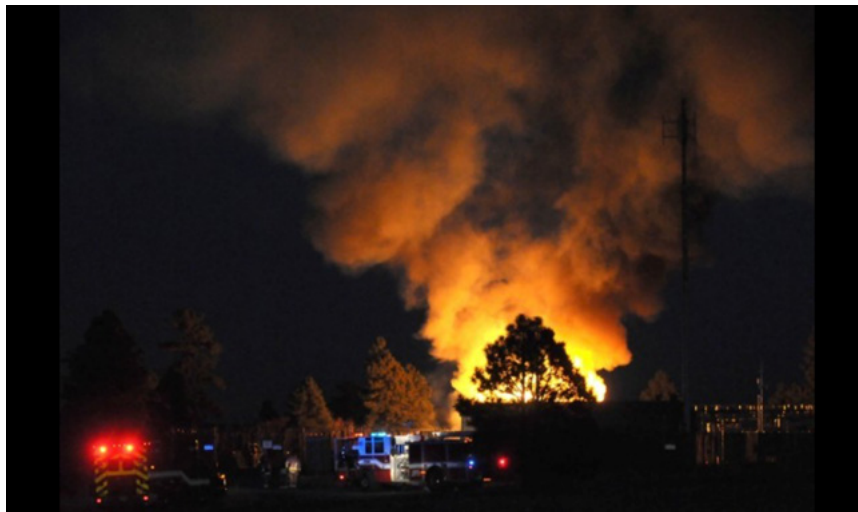
Figure 19 The 2012 BESS electrical fire at the Arizona Public Service facility near McMillan Mesa (Josh Biggs/ Arizona Daily Sun)
