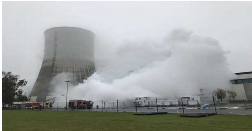
Figure 22. 2017 fire at an Engie Ineo BESS facility in Belgium (IMIA Report Photo)
